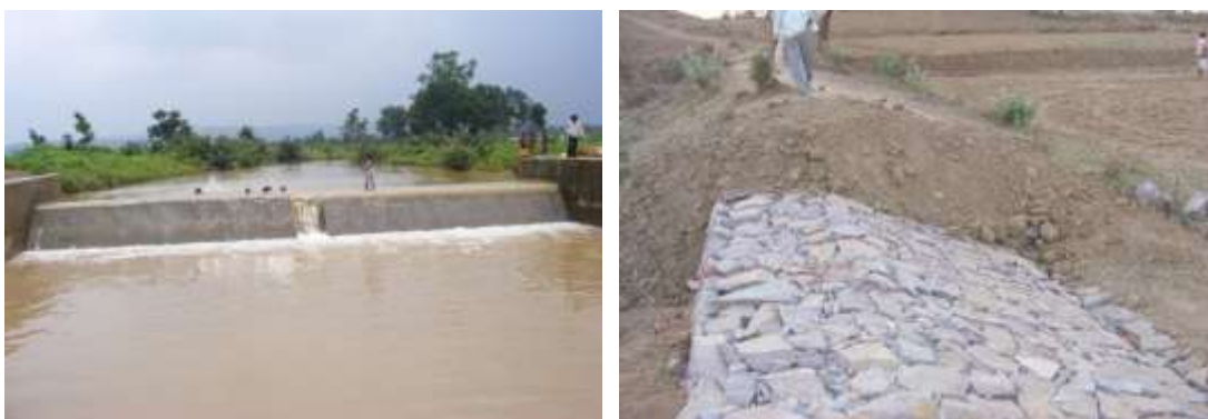
Fig 8: Ex-situ measures – check dam and gully plug
