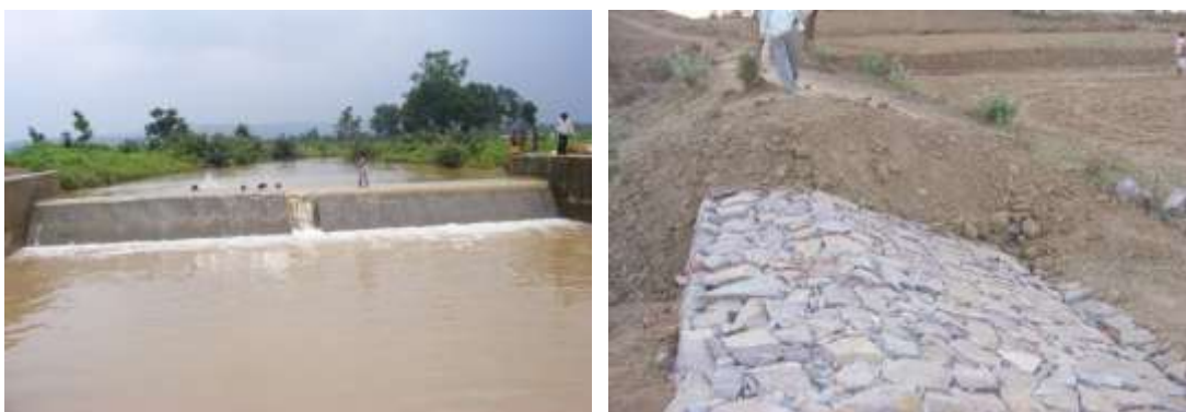
Fig 8: Ex-situ measures – check dam and gully plug
