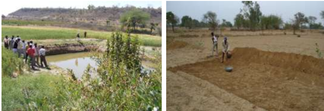
Fig 7: In-situ measures - farm pond and bunding
