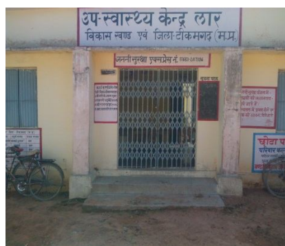
Figure 18 : The closed sub health center in Lar Khas village
