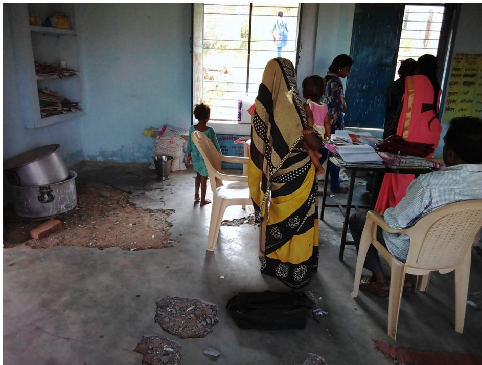
Typical anganwadi interior: damaged flooring, no place for play, no separate cooking or food storage area
