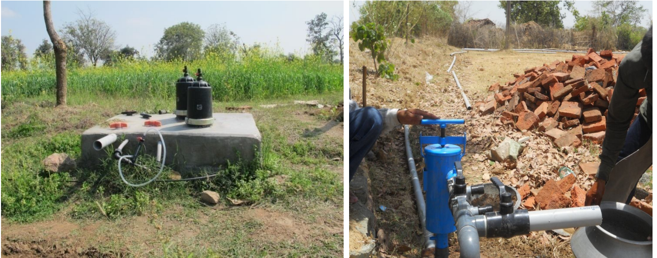
Pic 3.1: Main components of the drip irrigation system (before installation of main pipe and emission tubes)
