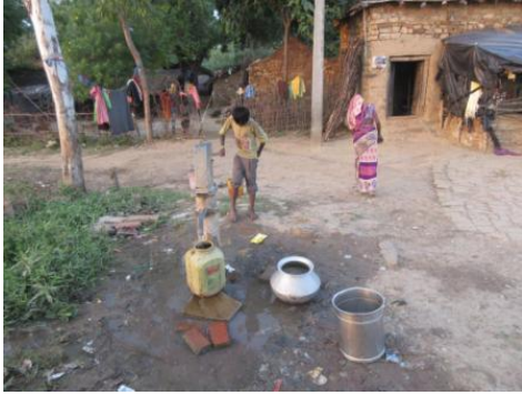
Handpump without platform
